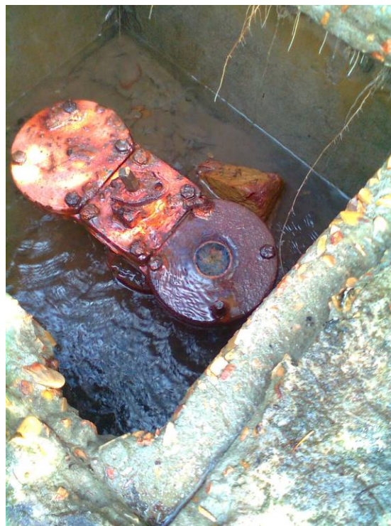
Figure 7: Leak on an airvalve on rising main to Kruisfontein
