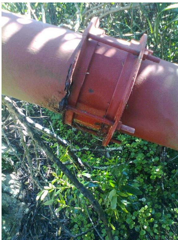
Figure 10: Leaking VJ coupling on the rising main to Kruisfontein
