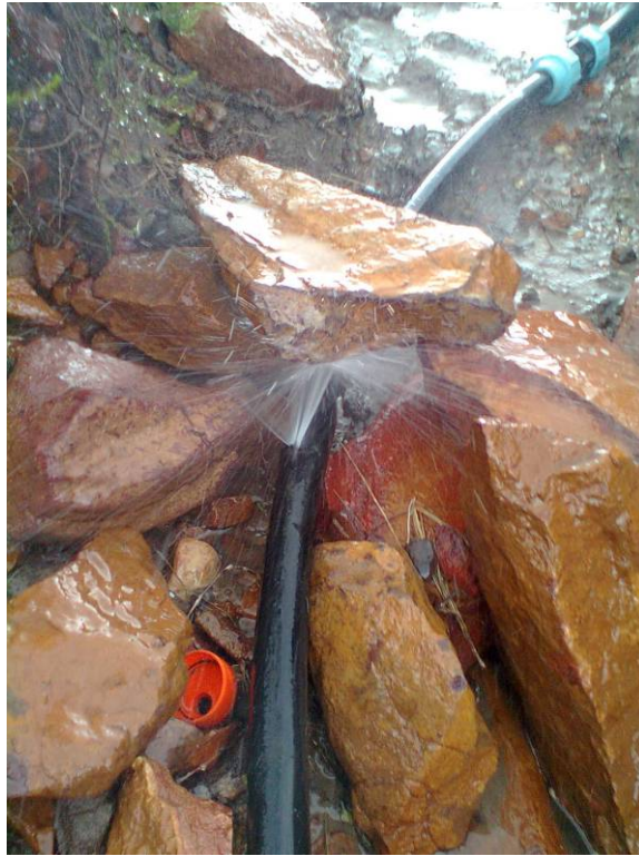
Figure 6: Another leak found on HDPE pipeline
