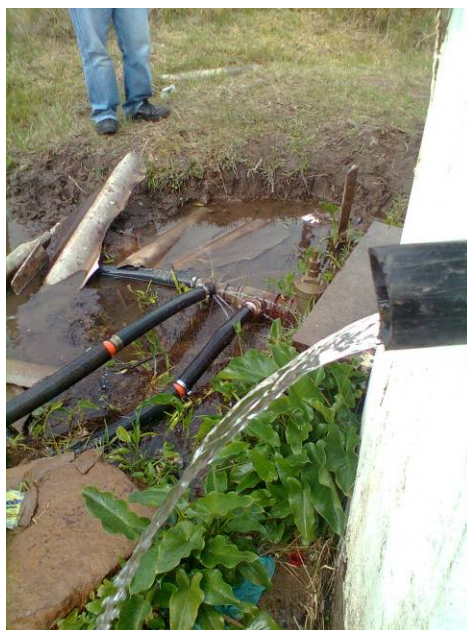
Figure 1: Overflowing reservoir with leaking outlet pipes
