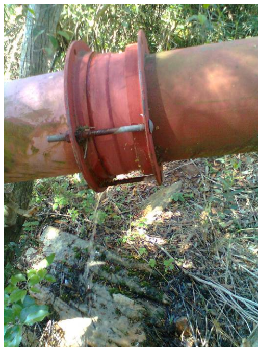
Figure 11: Another leaking VJ coupling on Kruisfontein rising main
