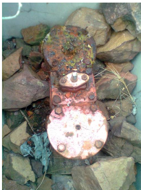
Figure 2: Damaged airvalve
