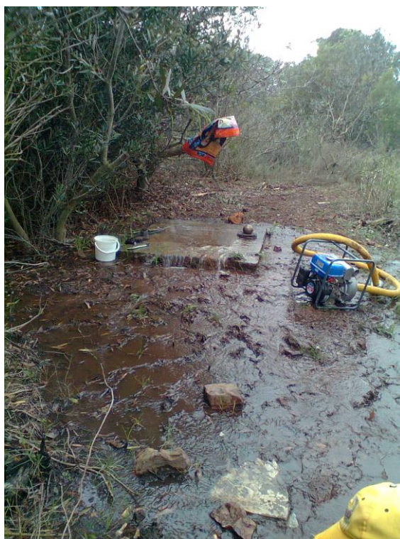
Figure 8: Another badly leaking airvalve on rising main to Kruisfontein
