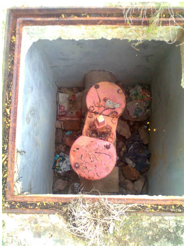
Figure 3: Another damaged air valve
