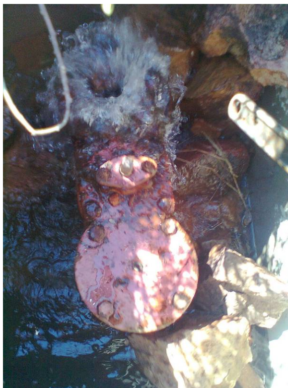
Figure 9: Another leaking airvalve on Kruisfontein rising main
